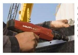
Powder-actuated tools should not be used in areas where flammable or combustible atmospheres may be present – the tool is a source of ignition and could cause an explosion. In these environments this process would be controlled by a permit to work system. The work would be regarded as **Hot Work** and would require high levels of focused safety management /supervision.
